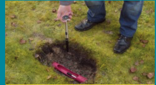
The sonde can be positioned very precisely and it helps to avoid extensive trenches.
