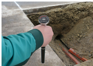
Tracing underground cables
